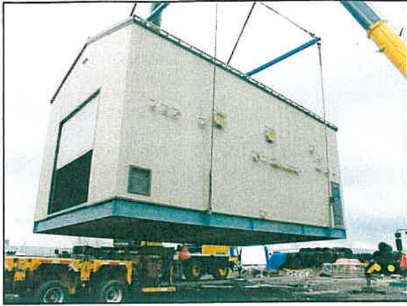
■ At an SAGD facility near Fort McMurray, Alberta, a VRU has been provided with a building to protect the equipment during cold weather. In winter, temperatures can be as low as -40°F (-40°C) for weeks at a time. This unit is rigid enough for a four-point lift to move the unit into position.
